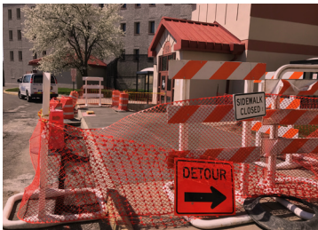
NYS Thruway Authority $1,300,000 Wallkill, NY
